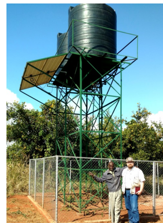
Jason and Pastor Paulino at Macate's new water tower
