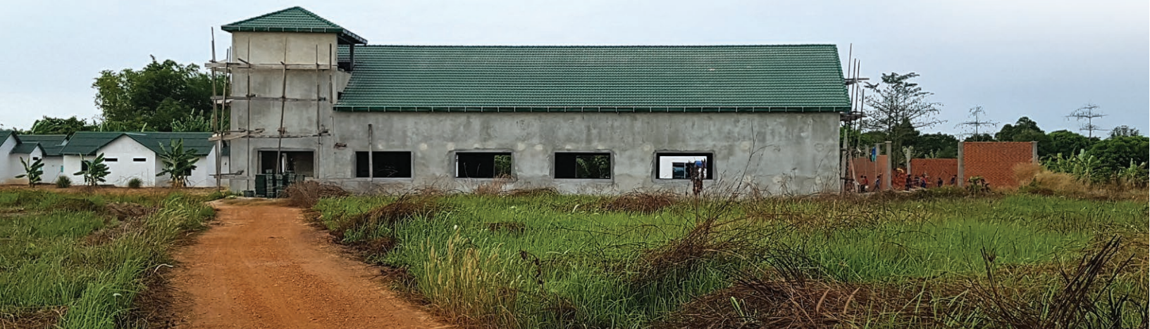
The new chapel building nears completion
