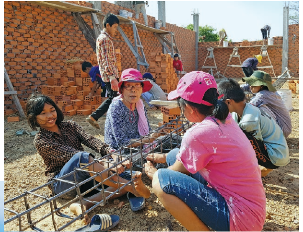
Working on the barn
