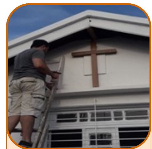
Moving, cleaning, fixing and reforming the new church building.
